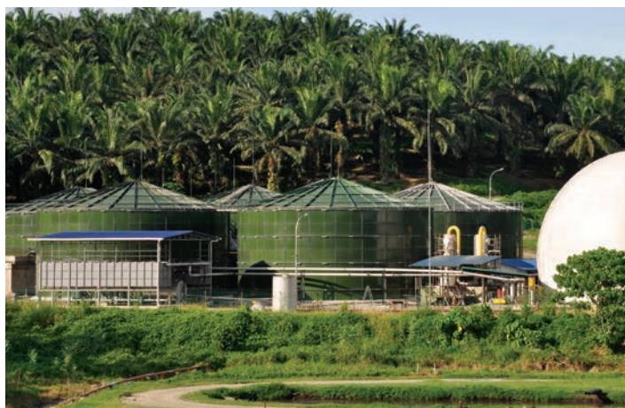
Commission of the two biogas plants in Pukin Palm Oil Mill, Johor (top) and Ladang Sabah Palm Oil Mill, Sandakan (bottom) to capture and mitigate GHG emissions.
