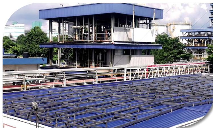
Solar thermal system under installation at IOI Pan-Cen for preheating boiler feed water
