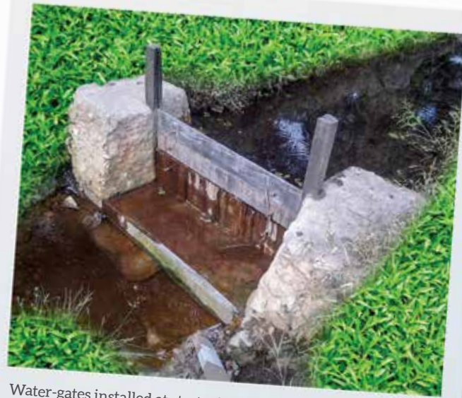
Water-gates installed at strategic locations to keep the water table at an optimum level
