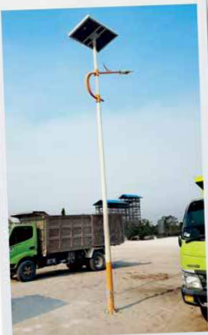
Solar street-lamp installed at IOI operation in Indonesia
